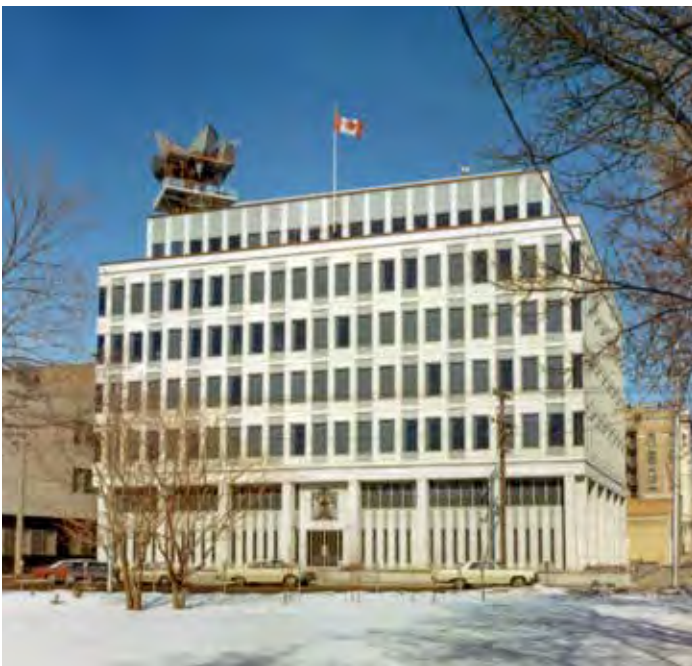
Built in 1962-63, the Bank of Canada building, as it appeared in the 1960s, was designed collaboratively by the Montreal-based architectural firm of Dunford, Bolton, Chadwick & Elwood and the local firm of Storey & Marvin. Flexman, Ruby (City of Regina Archives CORA-C-0891)
