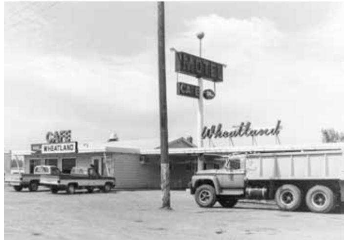
The Wheatland Motel, as it appeared circa 1980, located along the Trans-Canada Highway, just east of the ring road bypass. (City of Regina Archives CORA-A-0898)
