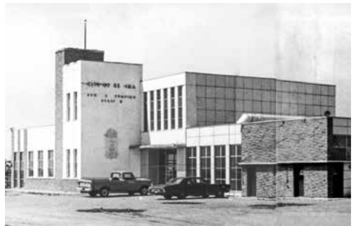
The City of Regina's sewage pumping station, located at 1010 McCarthy Boulevard, as it appeared in the 1960s. (City of Regina Archives CORA-A-1732)
