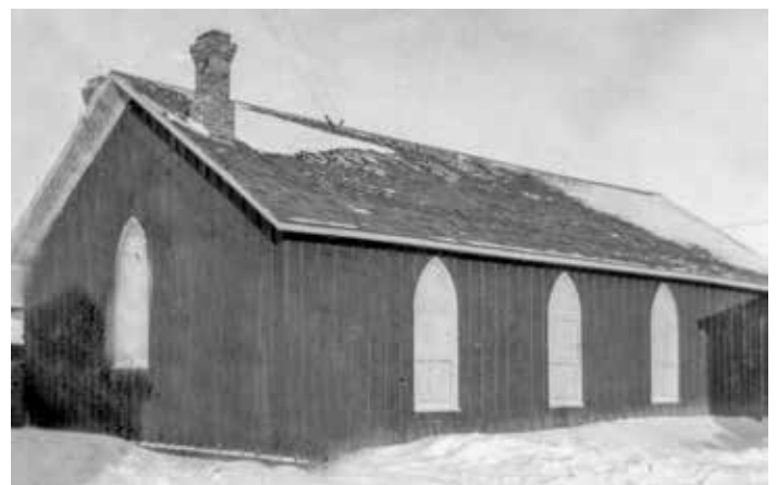
The first Anglican Church in the city, built in 1883 and formerly located at the corner of Smith Street and 12th Avenue. (City of Regina Archives CORA-B-0291)
