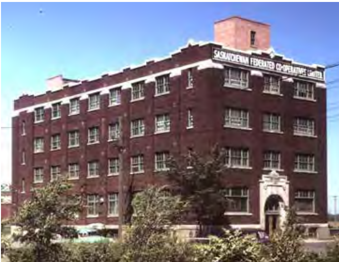
The Downing Building at 1150 Rose Street as it appeared in 1949. Built in 1914 and designed by Storey & Van Egmond for W.G. Downing and Co., the building was purchased by the Saskatchewan Federated Co-operatives Ltd. in 1943. Baker, Everett ( Saskatchewan History & Folklore Society SHFS 5867 2-X4 )
