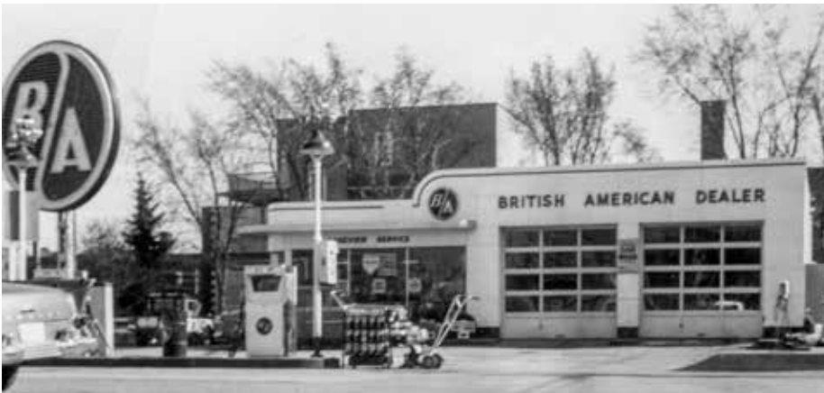
Lakeview Service Station at the southwest corner of Albert Street and 15th Avenue in 1964. (City of Regina Archives CORA-A-0182)
