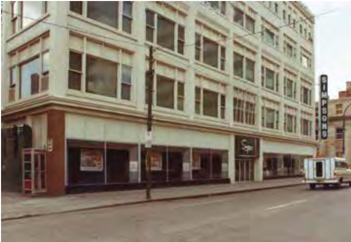
Formerly the R.H. Williams & Sons Department Store, purchased by the Robert Simpson Co. (later Simpson-Sears) in 1946, this large commercial edifice was demolished in the early 1980s. Located at the southeast corner of 11th Avenue and Hamilton Street. Caron, Lucien (City of Regina Archives CORA-C-2360)
