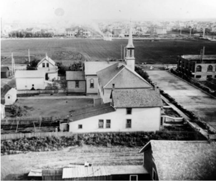
Located adjacent to St. Mary's Roman Catholic Church, fronting Cornwall Street just north of Victoria Park, St. Mary's (Gratton) School was the first purpose-built Separate School in the city, opening in 1900. Classes at the school ended in 1908. (City of Regina Archives CORA-B-0461)
