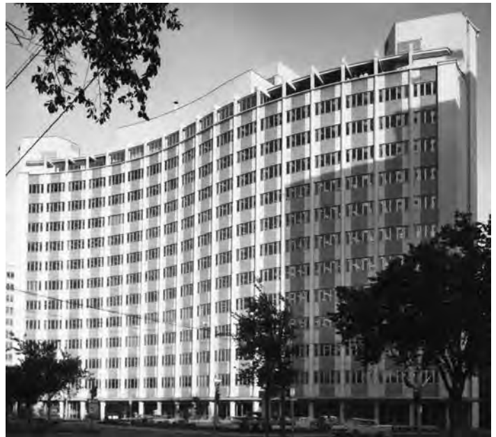
Designed by local architect Joseph Pettick, the Saskatchewan Power Corporation building opened in 1963. (City of Regina Archives CORA-B-0349)
