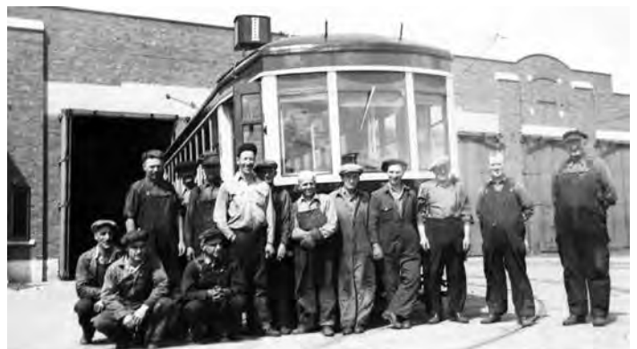
Maintenance crew in front of a Regina Municipal Railway streetcar at the car barns in the mid 1940s. The car barns would burn down later in the decade, with streetcar service ending a year later in 1950. (City of Regina Archives CORA-A-0465)
