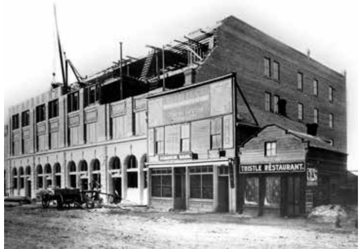
The King's Hotel under-construction along Scarth Street, north of 11th Avenue. (City of Regina Archives CORA-B-0300)
