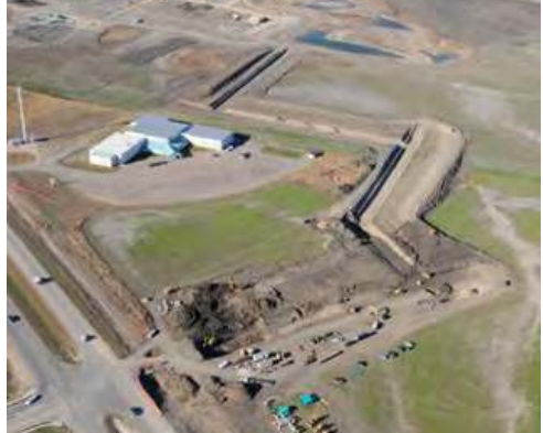
Photo: Area grading shapes the future residential blocks, parks, and roads.
