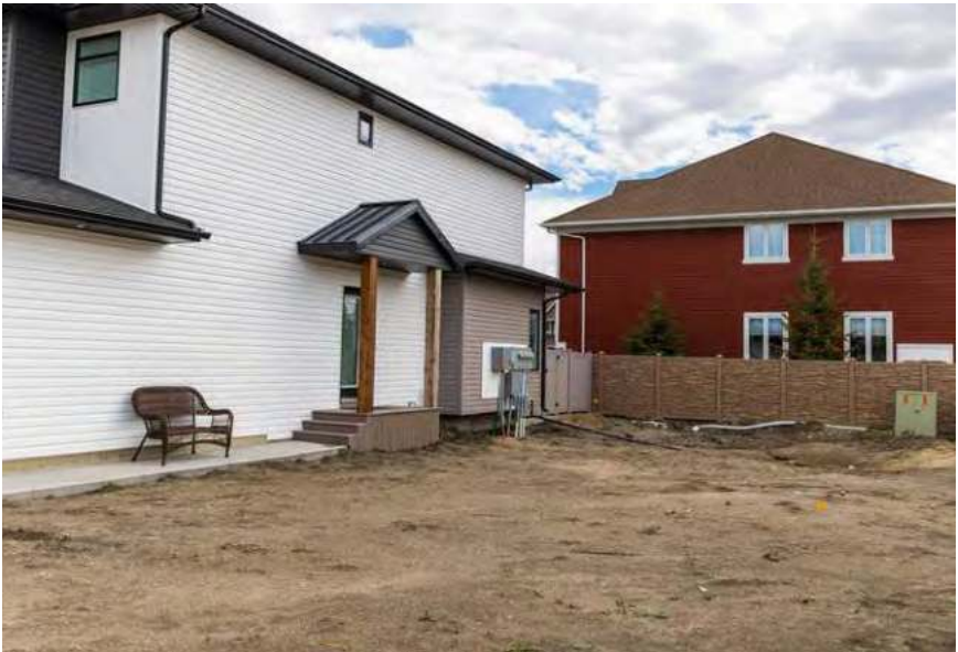
Photo: Proper Lot grading protects your home from basement flooding and other drainage issues.
